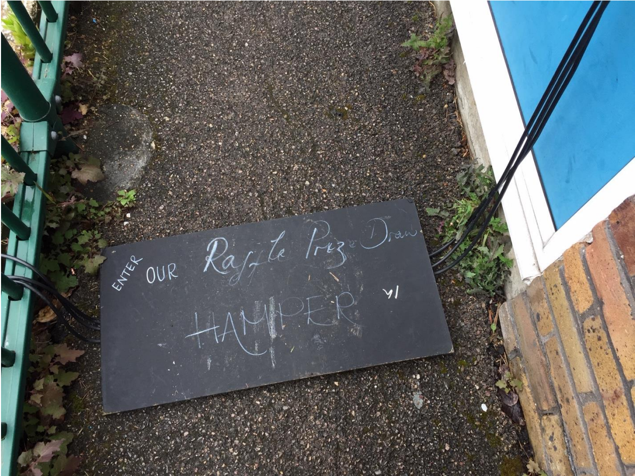
Cable covered with blackboard increasing the hazard of tripping on this
